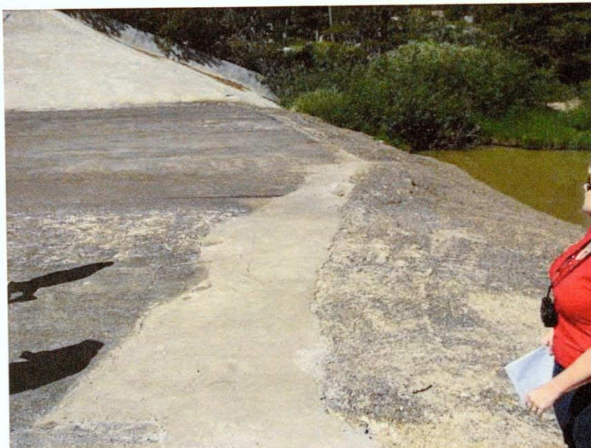
2. Close up view of the downstream end of the notched section (at the hinge point), showing the repairs made to the concrete invert slab last year.
