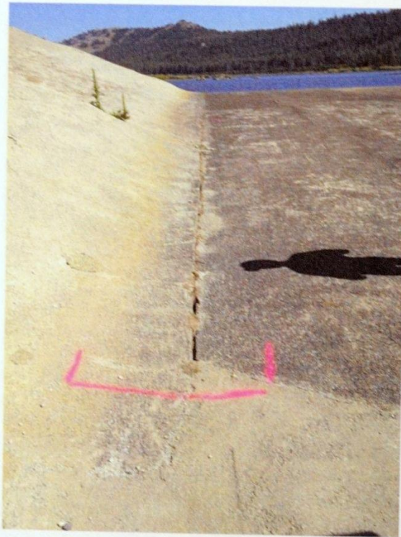
Photo 4 – Painted area to be cut and filled with concrete.
