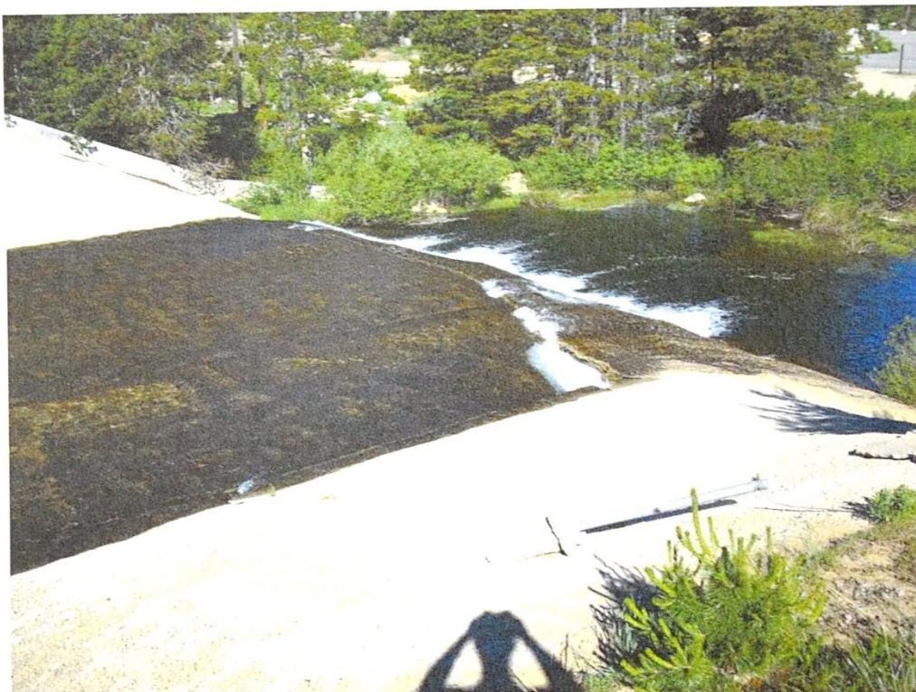
4. Crack in downstream end of spillway apron causing leakage.
