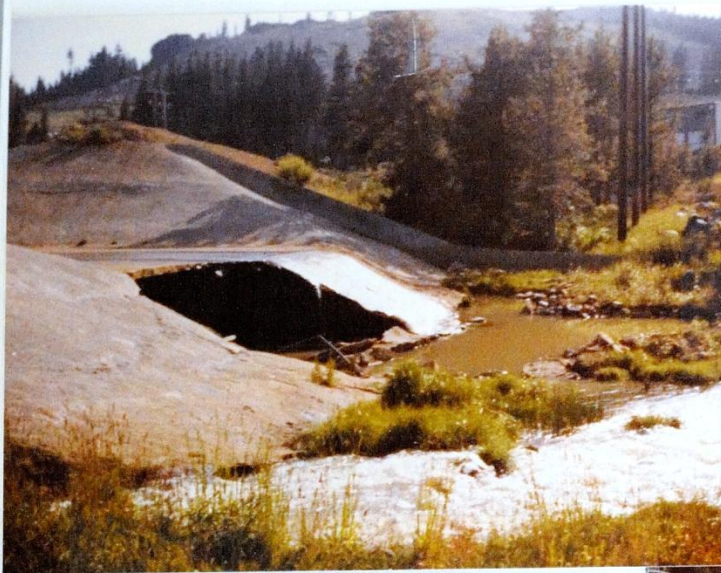
Failure of New Spillway
