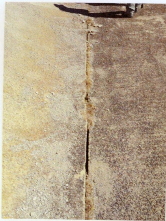
Photo 3 – Cold joint void between right abutment and spillway
