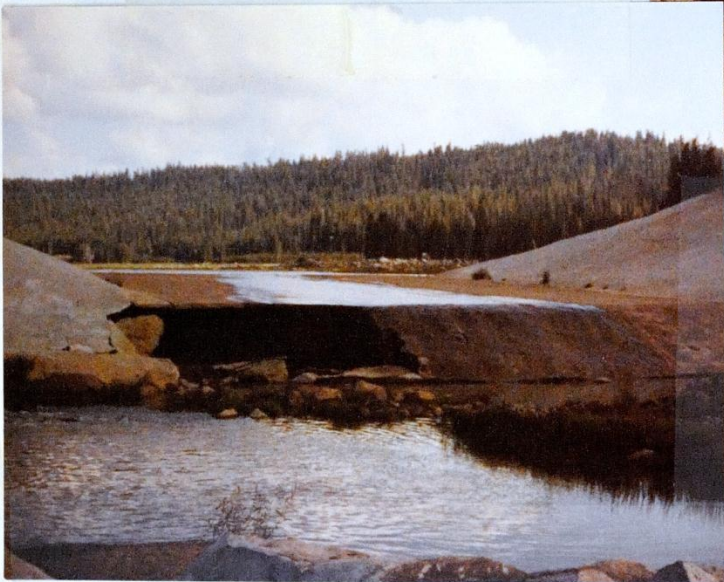
Failure of downstream end of the new spillway.
