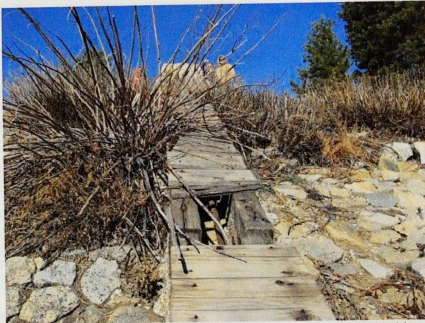
9. The outlet stem in a timber trunk on the upstream face, looking upslope.
