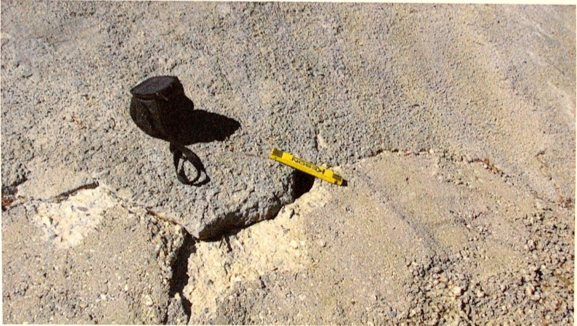
5. Close up view of the spalled and cracked concrete at the downstream end of the spillway.
