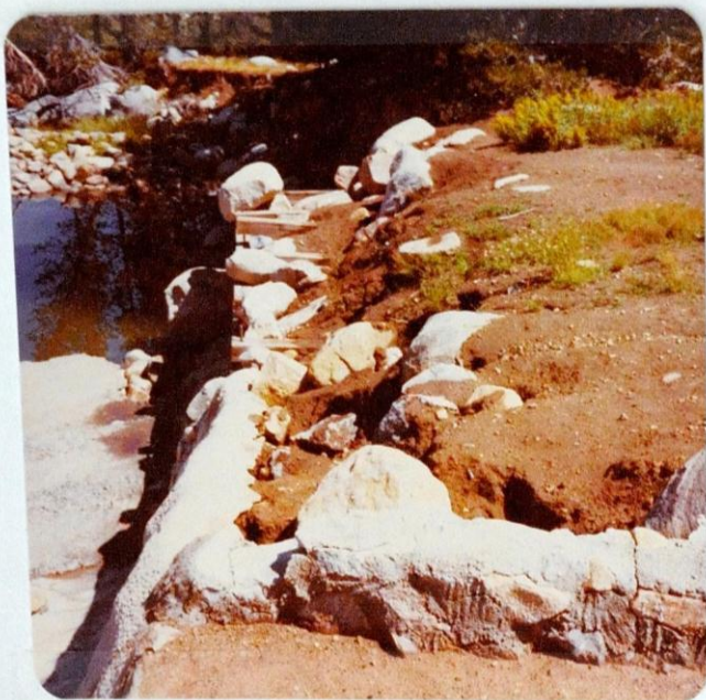
Surface erosion on top of right spillway wall.
