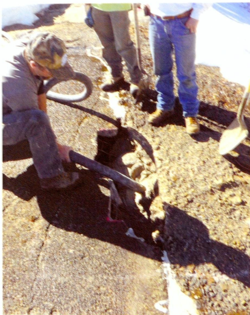
Photo 1 – Pumping concrete into large void near the end of the spillway.
