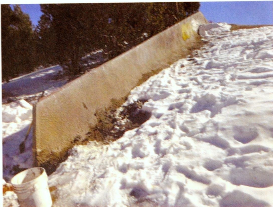
Photo 5 – Hole cut on top of spillway to fill void in Photo 6 location
