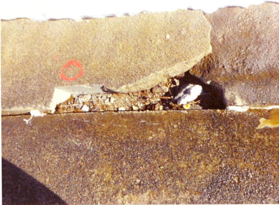
Photo 2 – Small void that was sawcut
