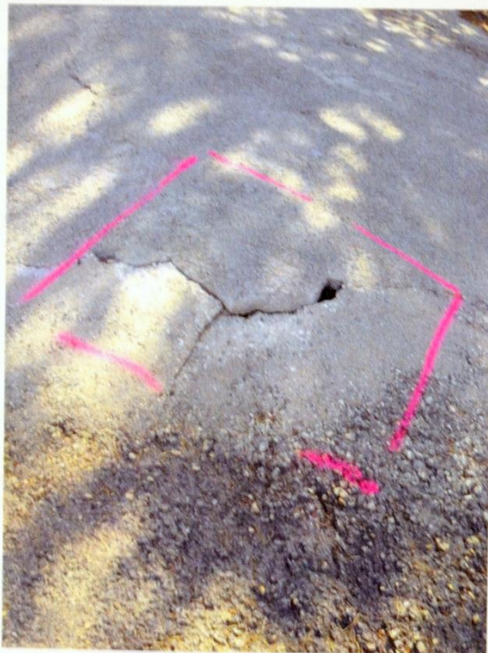
Photo 6 – Void along spillway and left abutment to be cut and filled with concrete.
