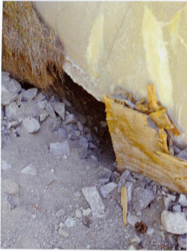
Photo 1 – Void under spillway, right abutment
