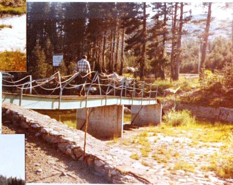
Snow load from adjacent road collapsed end section of old spillway walkway.
