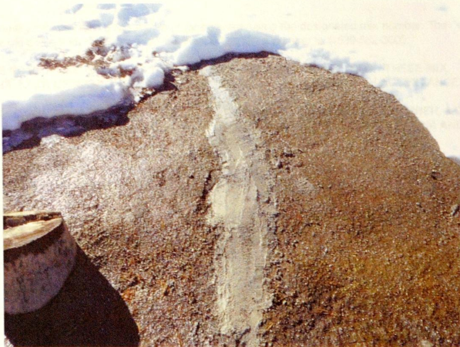
Photo 7 – Finished patch on left abutment of spillway.
