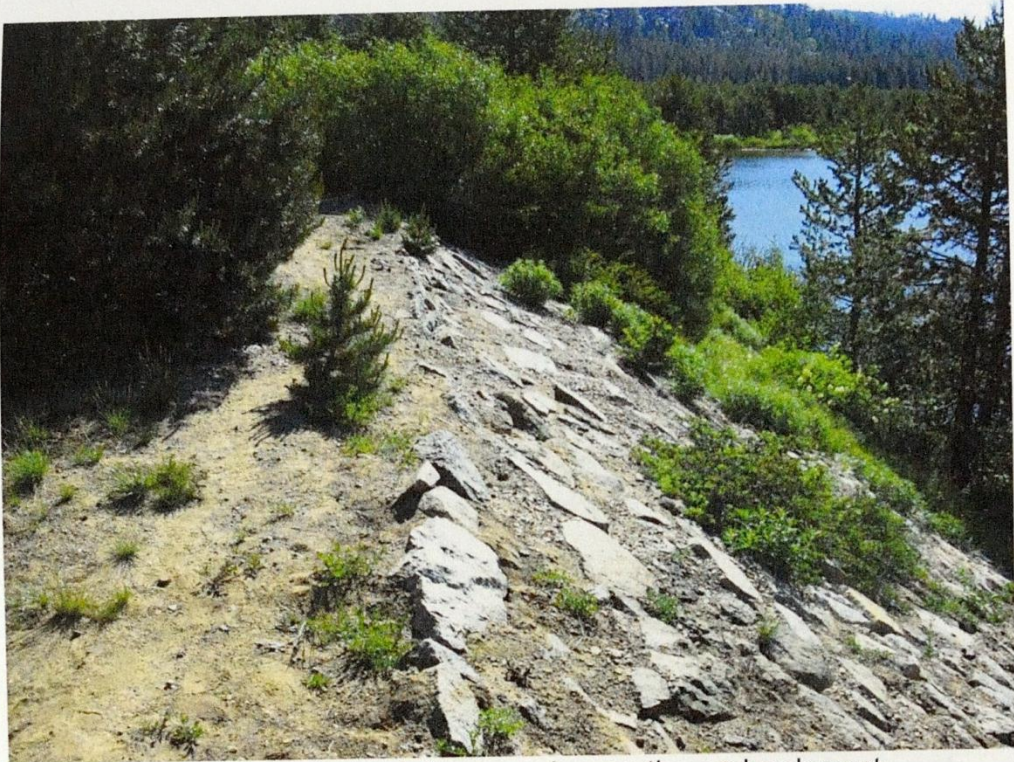
5. Typical vegetation growing on the embankment.
