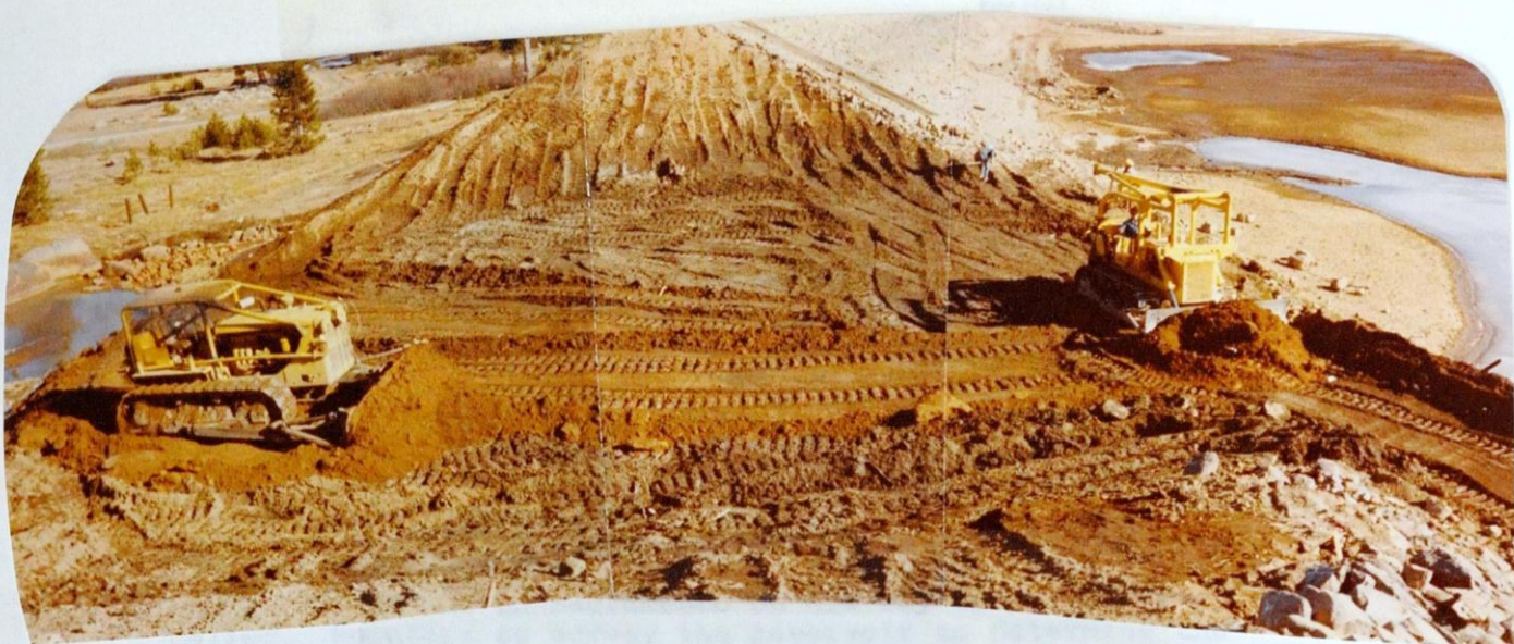
Excavation for breach of dam at approximately Elevation 6750.
