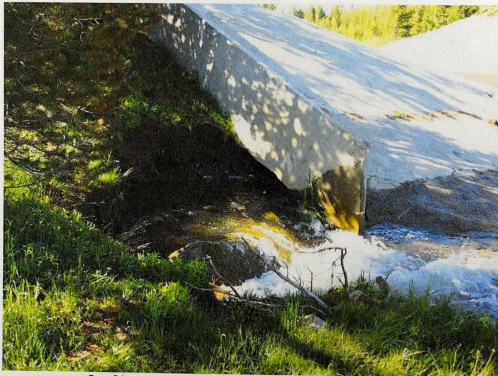
2. Close-up of water coming under spillway lining.
