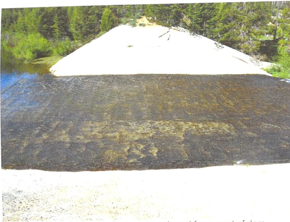
3. Gunitite-lined spillway apron viewed from crest of dam.
