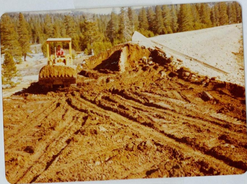
Breaching embankment.
