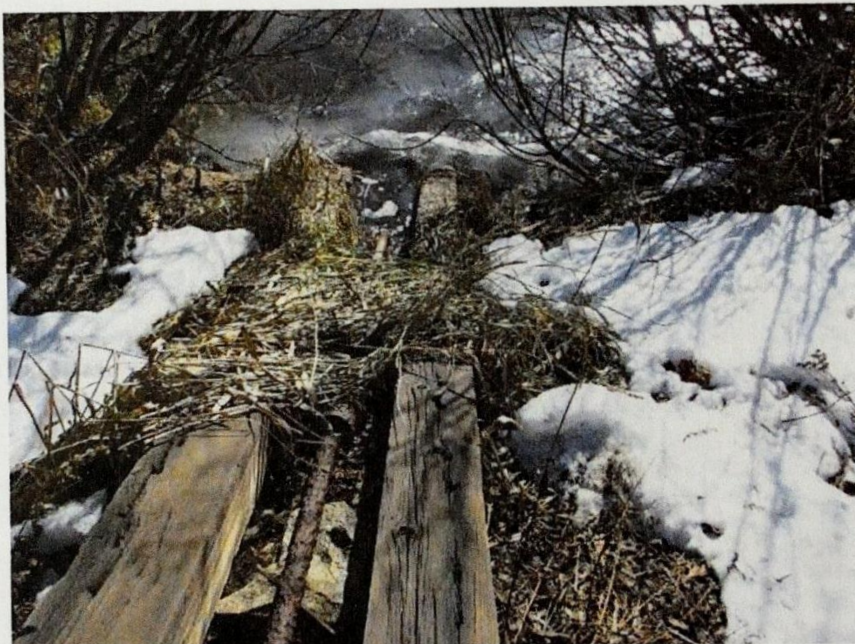
10. The rusted outlet stem, looking downslope. The outlet gate is in the closed position and has not been cycled in decades. Its operability is doubtful.
