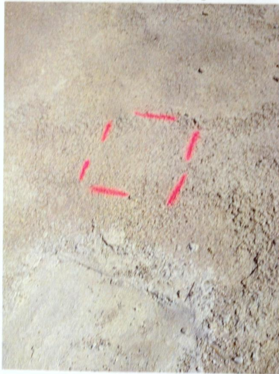
Photo 2 – Area to be cut in spillway above void in Photo 1.
