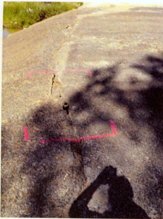
Photo 5 – Hinge point on spillway to be cut and filled with concrete.
