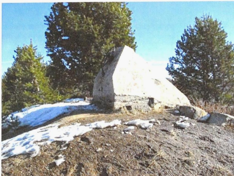
11. The outlet gate concrete pedestal and handwheel, located on the crest to the right of the notched section. Matures trees in the background are present all over the embankment.
