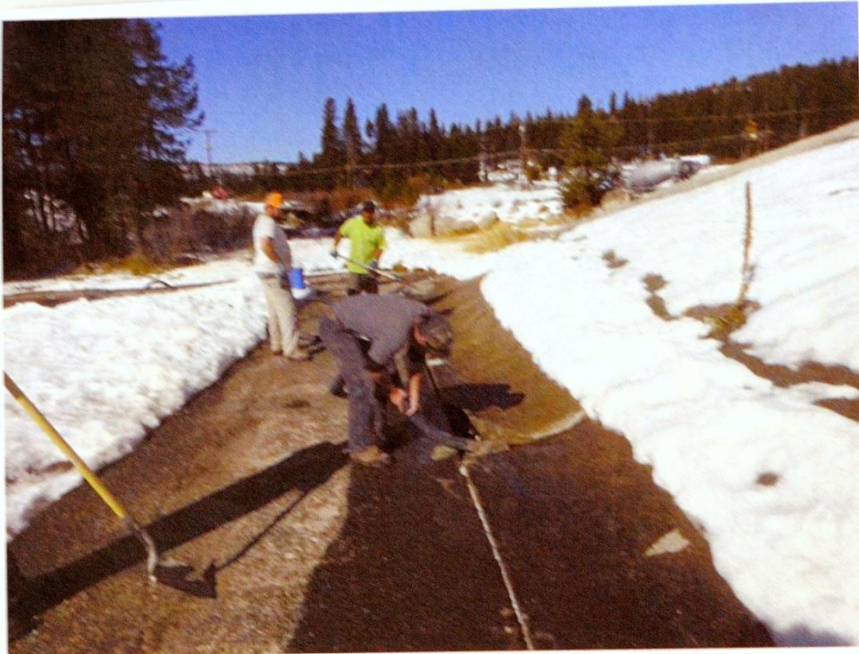
Photo 4 – Concrete filling of transverse crack
